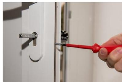
**7. Step – Attach the cylinder on the outside**
