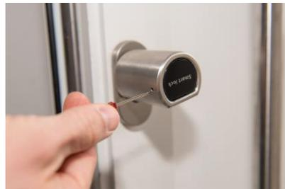
**8. Step – Attach the cylinder on the inside**
