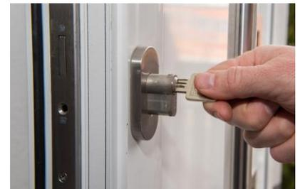
Now you can push the FLEX fingerprint cylinder through the lock, from the outside to the inside. **Pay attention that the fingerprint handle is on the outside of the door.** When the cylinder is attached to the door you need to screw down the cylinder as shown in the 2 pictures below.
