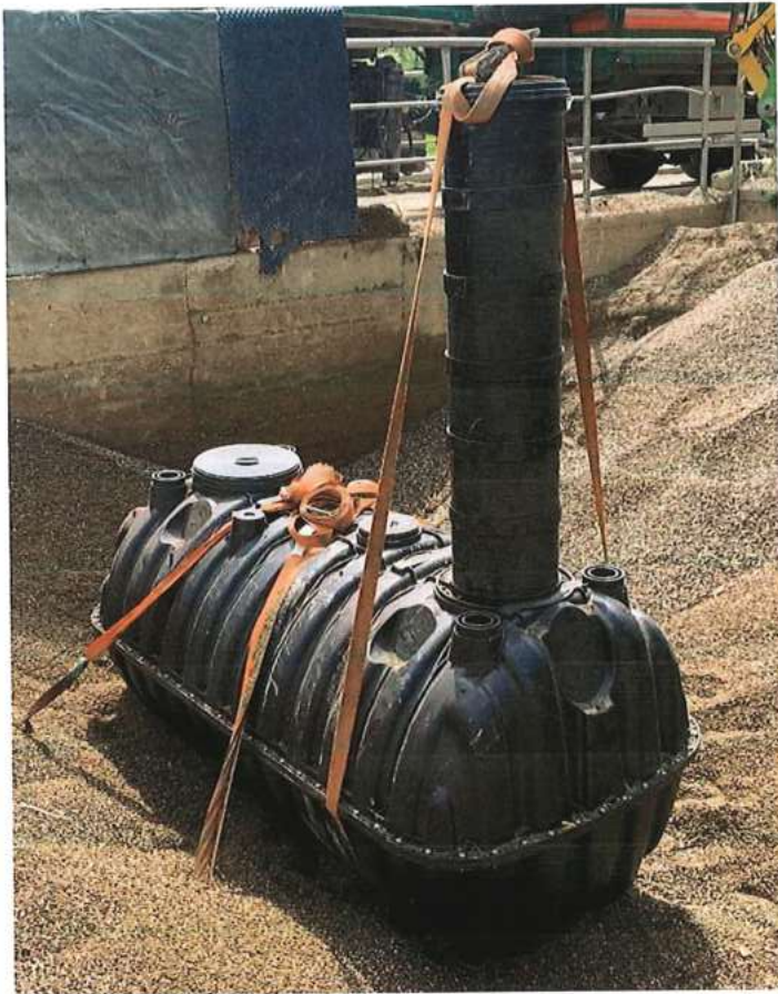
Figure 2: Tank placed in pit
