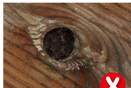
Knot holes – not permitted from 10 mm
