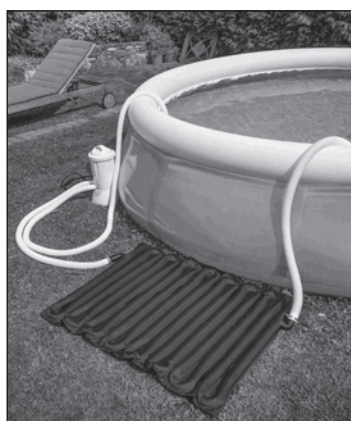
Solar Pool Water Heating
